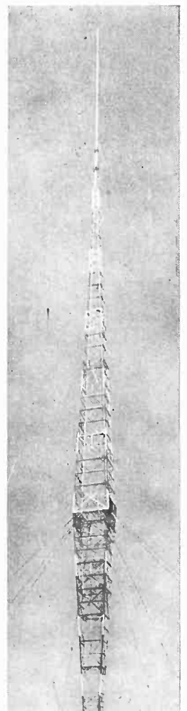
WLW's double-taper tower. Increases in signal strength up to 40% were reported when it was installed.
